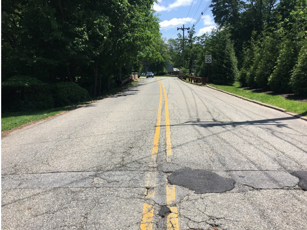
View looking easterly at Morris County Bridge on Sunset Road.
