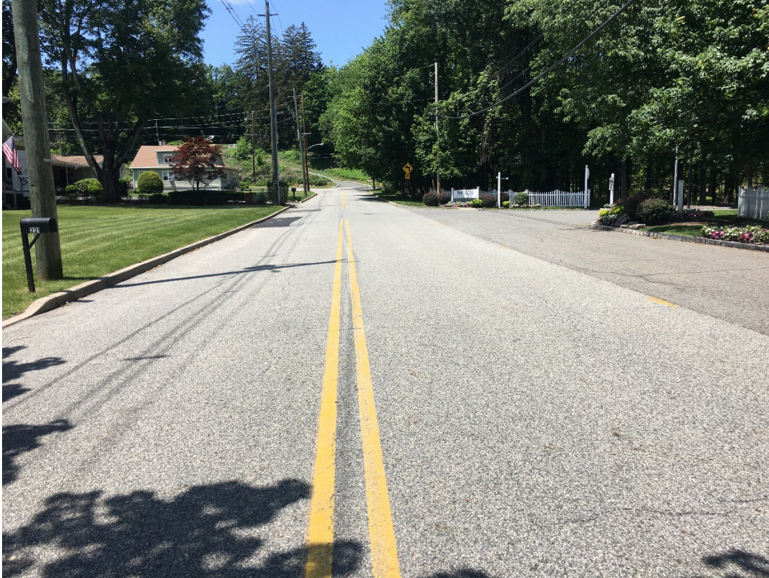
View looking westerly down Sunset Road across 'The Glens' development main access
