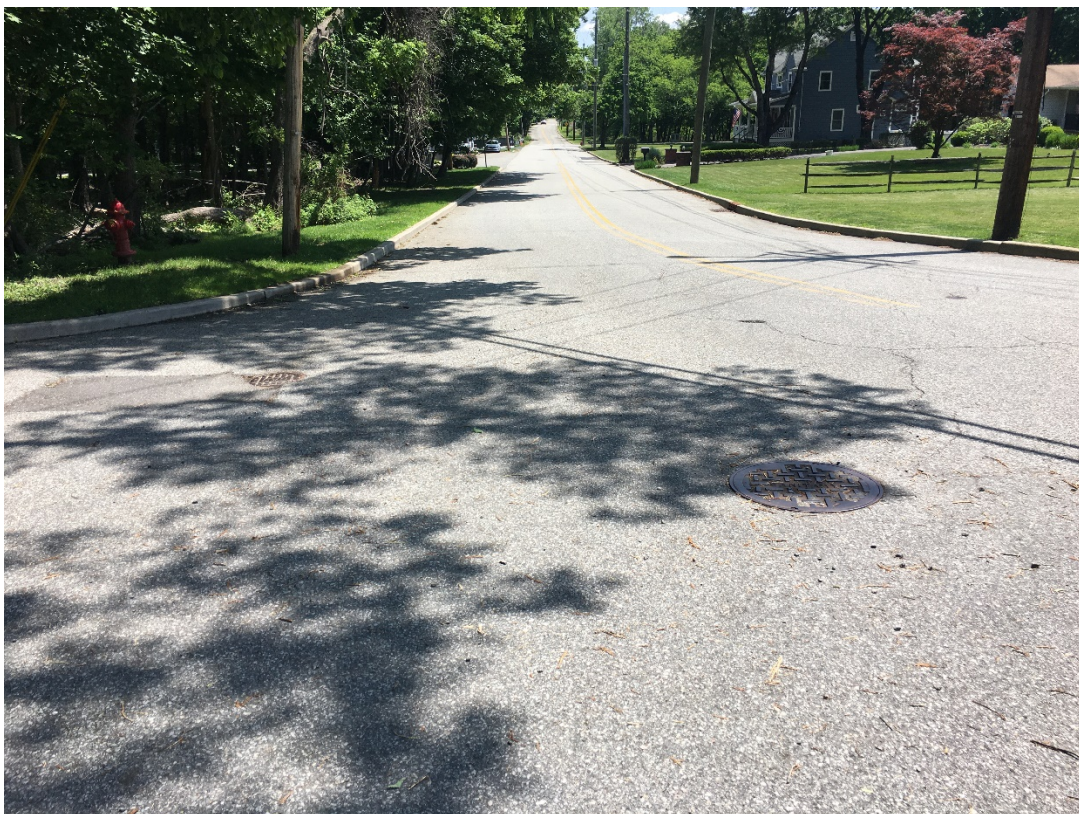
View looking easterly up Sunset Road from West Sunset Road intersection.
