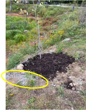
Figure 2a. Gravel-filled Gully
