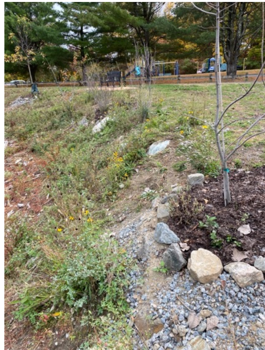
Figure 1b. Previously Installed Terraces: Still Good.
